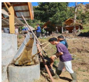
Gambar 2. Proses Pengisian Kohe Sapi ke Digester
